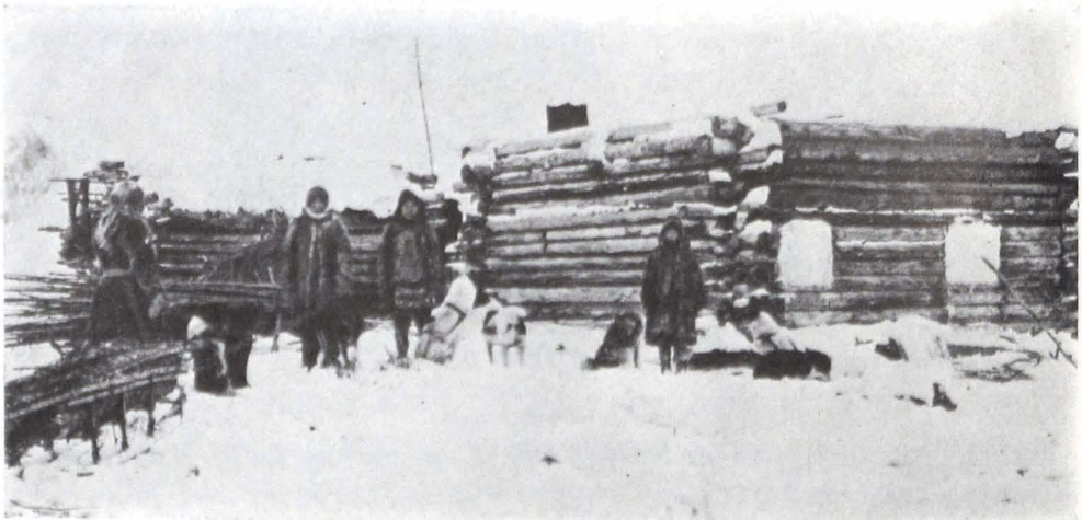
Fig. 45. A Flat-Roofed Blockhouse of the Upper Kolyma Yukaghir which serves as a Winter Dwelling. The windows are covered with thick panes of river ice.
