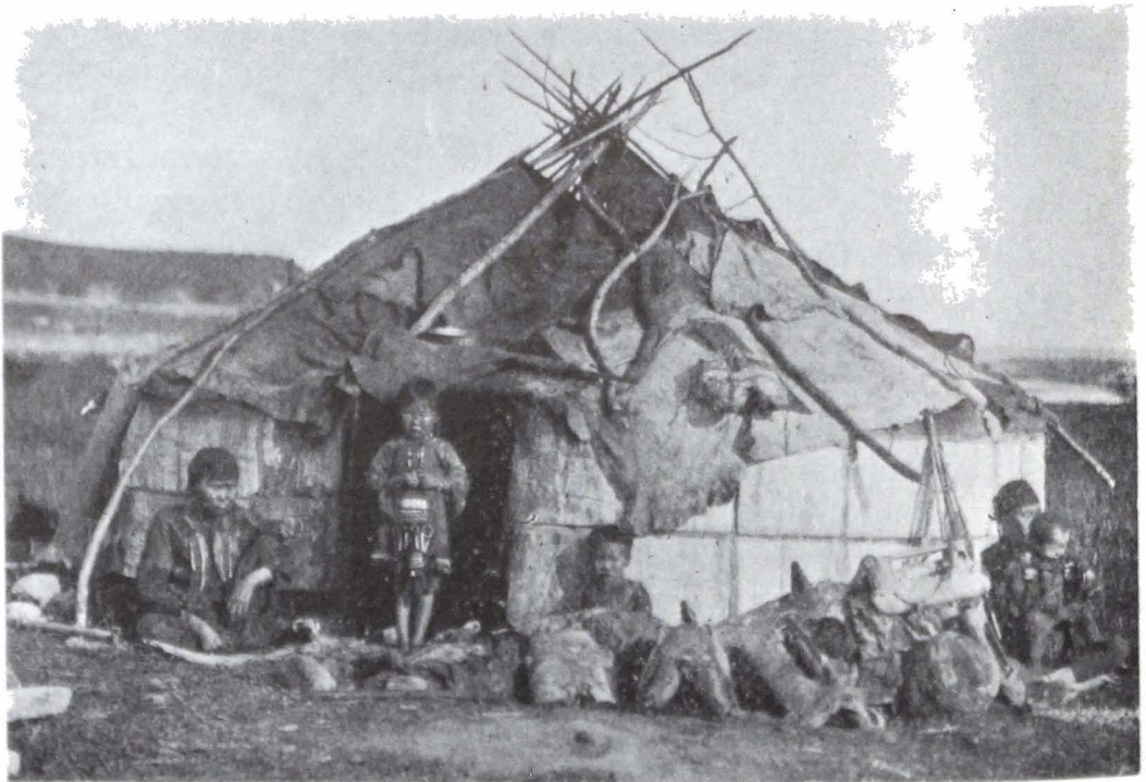
Fig. 39. A Cylindro-Conical Tent of the Okhotsk Tungus. The upper, conical portion, is covered with reindeer skins; the lower, cylindrical section, is of rectangular sheets of birchbark sewed together with thongs.
