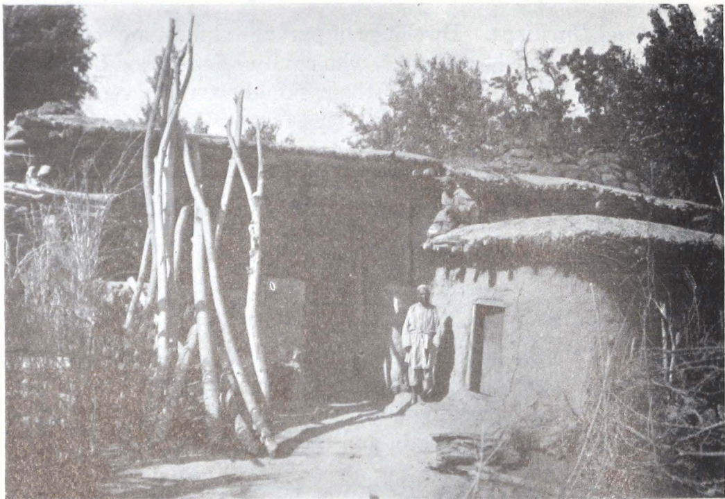
Fig. 46. Inner Court of a Tadjik Dwelling, Eastern Bokhara. The house is a flat-roofed structure made of mud and clay.
